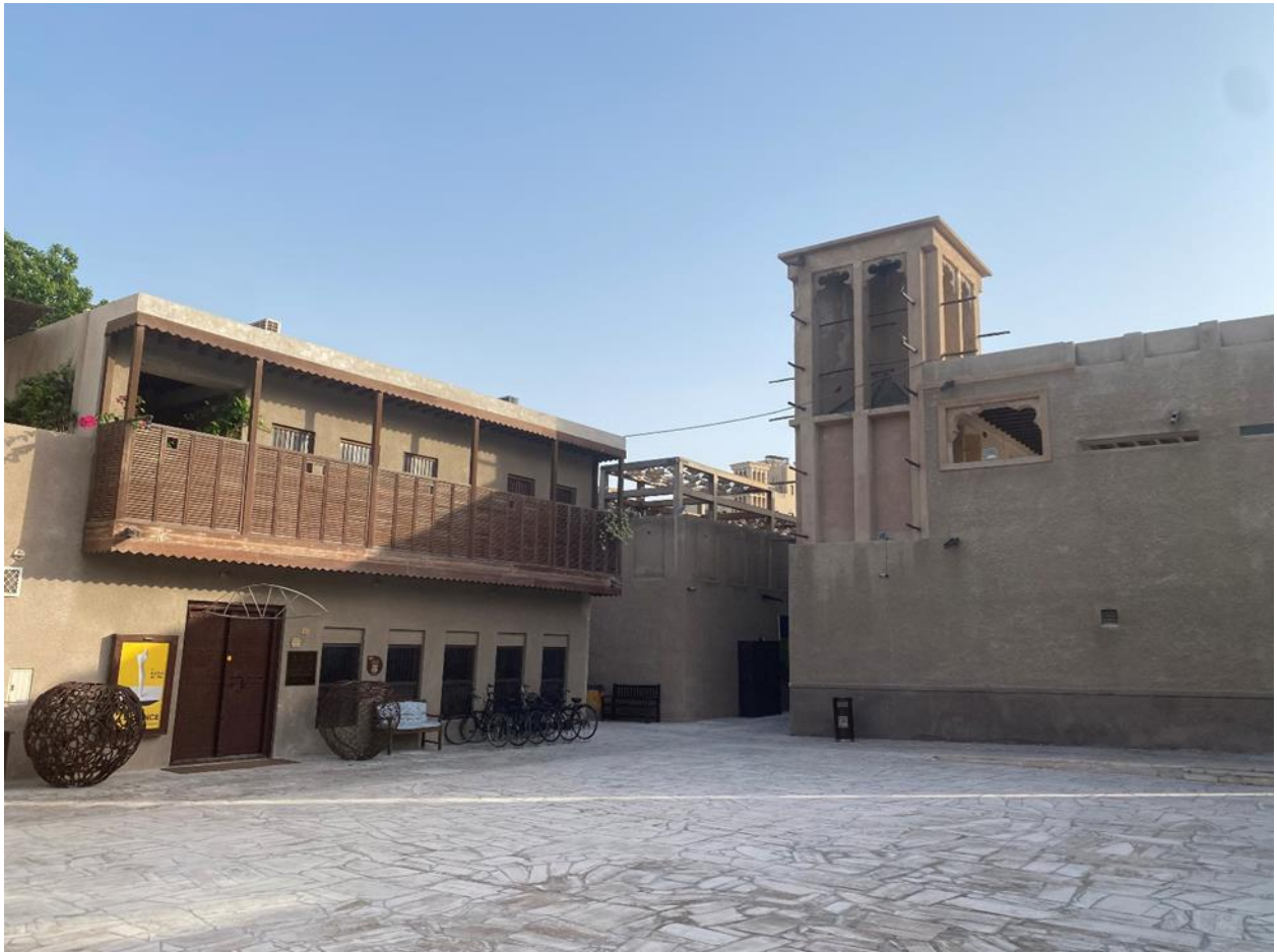
FIGURE 12: MASHRABIYAS'S DISTINCTIVE ARCHITECTURAL FEATURE, (TAKEN BY AUTHOR)
