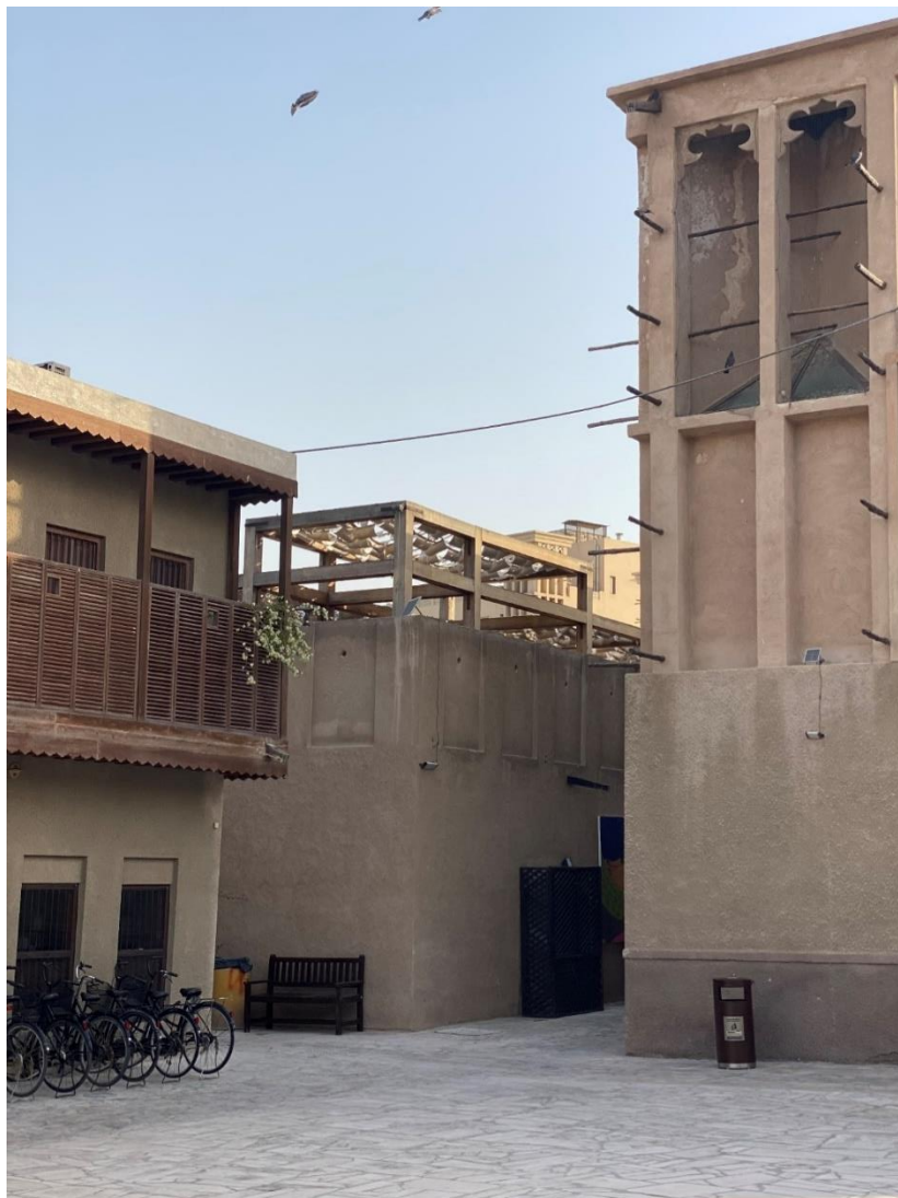
FIGURE 8: DISTINCTIVE ARCHITECTURAL FEATURES IS THE WIND TOWER, OR 'BARJEEL, (TAKEN BY AUTHOR)
