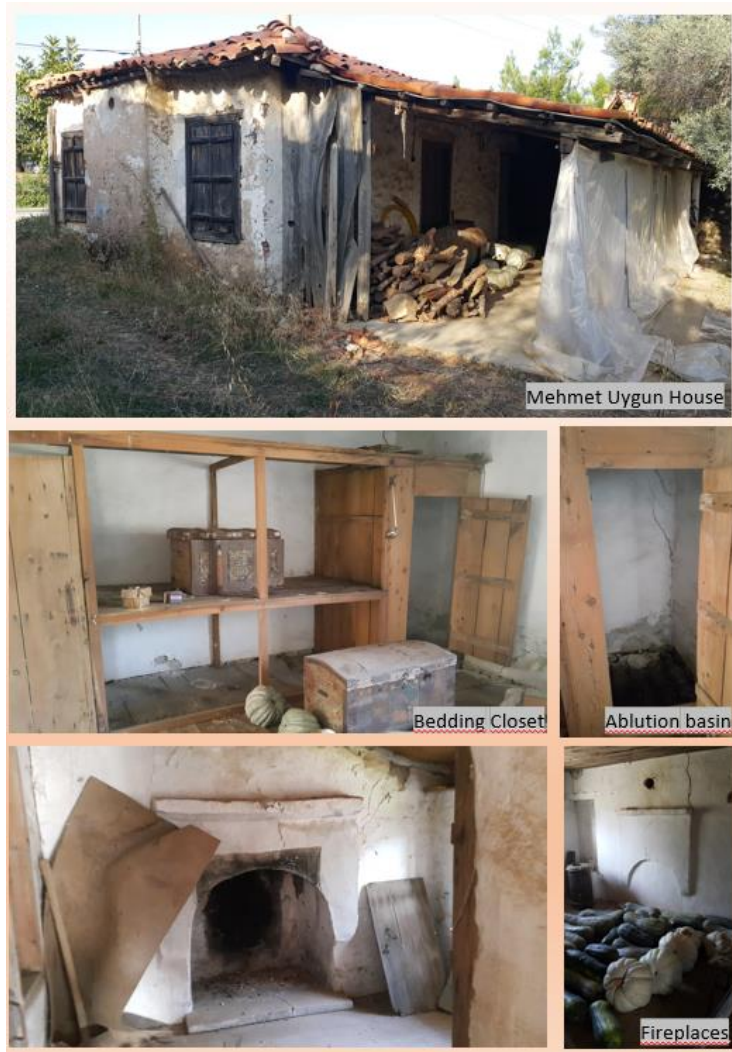
Figure 5. Mehmet Uygun House used as a storage
