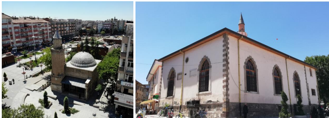
Figure 1. Hoca Hasan Masjid and Hacı Hasan Masjid (Photographs by the authors, 2019)
